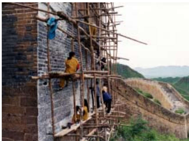
Working at the Great Wall
